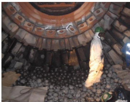
Lining areas rebuilt and protected
