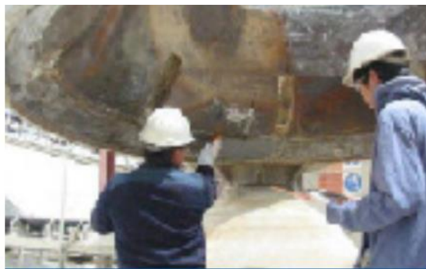
Rebuilding in progress
