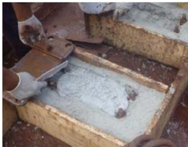
Restoration in progress
