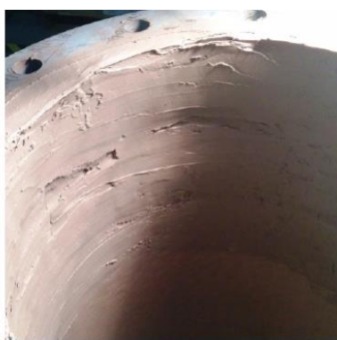
Internal surface rebuilt
